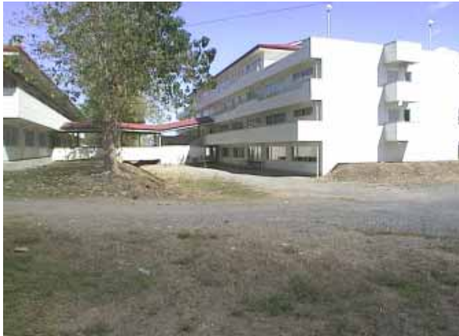
Figure 3. Dormitory and cafeteria facilities at PhilRice Headquarters
